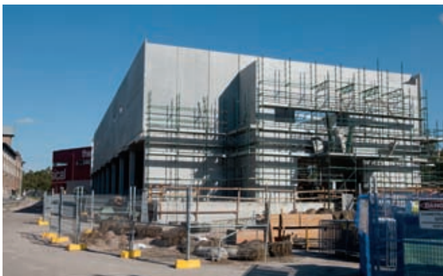
The Gallery's new Collection store in various stages of construction from January 2009.
